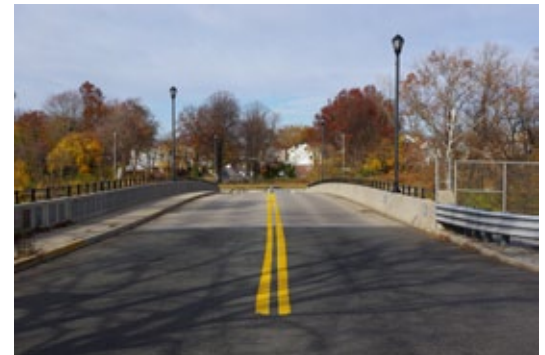
The Bridge Monument , 2010. Photo by Charles Harlan.
